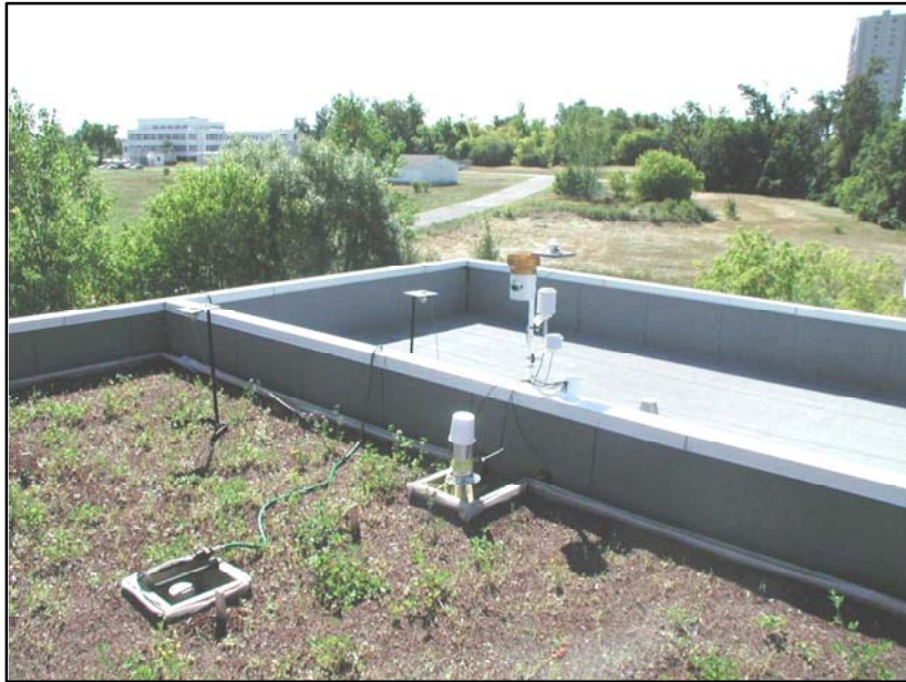
Figure 4.3: The Field Roofing Facility on the NRC campus in Ottawa, June 2001. The median divider separates the Green Roof (left) and the Reference Roof (right). A weather station is located at the median divider.
