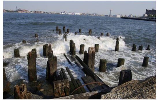
Detail of Reef, Day of installation at Low Tide (Pre-Oysters), June 2007
